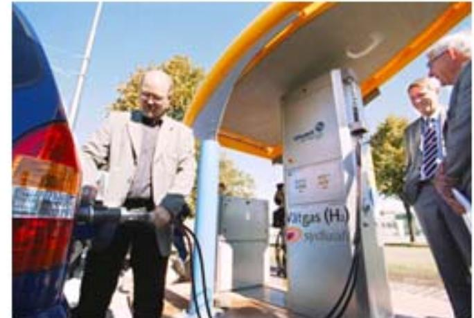
A hydrogen dispenser at a refuelling station in Sweden (source: Ludwig-Bolkow-Systemtechnik)
